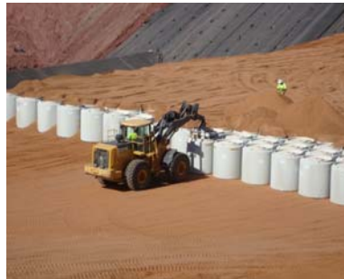
Waste Control Specialist's disposal of DOE byproduct waste from Fernald
